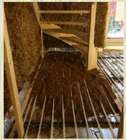
QuickTime<sup>®</sup> and a decompressor are needed to see this picture. Radiant floor heating
